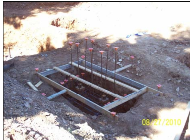
Figure 6: Dimensional Lumber Formwork at Top of Pile Cap
