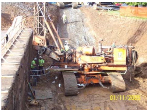
Figure 10: Steel Soldier Pile Installation at Existing Tunnel
